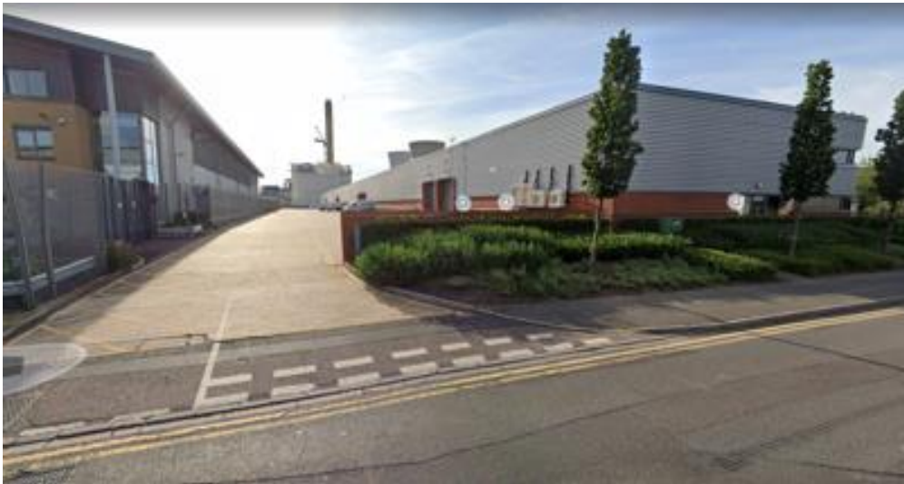
Plate 13.2 - View from Liverpool Road (220m east) view between gap of two buildings (baseline prior to demolition onsite).
