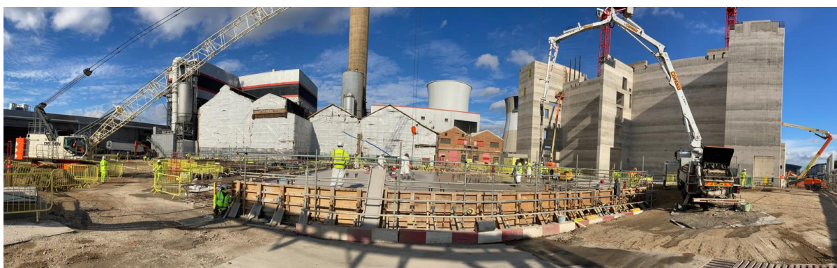
Plate 2.2 – Site Panoramic, Existing Consented Scheme, Boiler Hall foundations (Date: October 2021)
